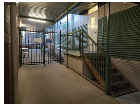
P4 PAVED WALKWAY & THE AWNING OVER TO BE RETAINED. FENCING AND SECURITY GATE, DEMOUNTABLE AND THE STEPS WITH THE AWNING ABOVE THE STEPS TO BE REMOVED
