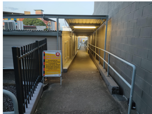
P10 PAVING TO BE DEMOLISHED IF ON GROUND, IF SUSPENDED RETAIN. RETAINING WALLS TO DEMOUNTABLE TO BE DEMOLISHED. RETAINING WALLS TO STORES BUILDING (BLOCK STRUCTURE) TO BE RETAINED. REFER TO STRUCTURAL DOCUMENTATION FOR DETAIL OF BLOCK WALL DEMOLITION FOR STORES EXPANSION.
