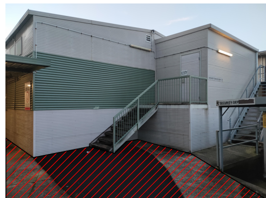
P7 HATCHED PAVING TO BE DEMOLISHED INCLUDING SIMILAR SURFACES UNDER DEMOUNTABLE ONCE REMOVED. NOT HATCHED PATH AND HANDRAILS TO BE RETAINED TO SECURITY OFFICE STAIRS.
