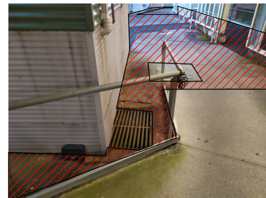
P5 HATCHED PAVING TO BE DEMOLISHED INCLUDING SIMILAR SURFACES UNDER DEMOUNTABLE ONCE REMOVED. NON HATCHED PATH AND HANDRAILS TO BE RETAINED.
