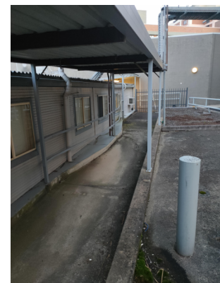
P8 PAVING TO BE DEMOLISHED IF ON GROUND, IF SUSPENDED RETAIN. RETAINING TO RHS TO BE RETAINED. TO LHS TO BE DEMOLISHED TBC WITH CIVIL & STRUCTURAL ENGINEERS. DEMOUNTABLE & AWNING STRUCTURE TO BE DEMOLISHED. REFER TO SERVICES ENGINEERS DOCUMENTS FOR CABLE TRAY TERMINATIONS
