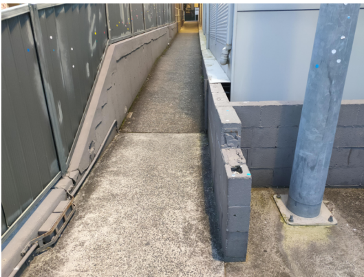
P14 RETAINING WALL LEFT SIDE ADJACENT TO LOADING DOCK TO BE RETAINED. PAVING TO BE DEMOLISHED IF ON GROUND. IF SUSPENDED RETAIN. RETAINING WALL ADJACENT TO DEMOUNTABLE TO BE DEMOLISHED. DEMOUNTABLE. TO BE REMOVED. LIGHT POLE RELOCATED TBC WITH SERVICES ENGINEERS DOCUMENTS
