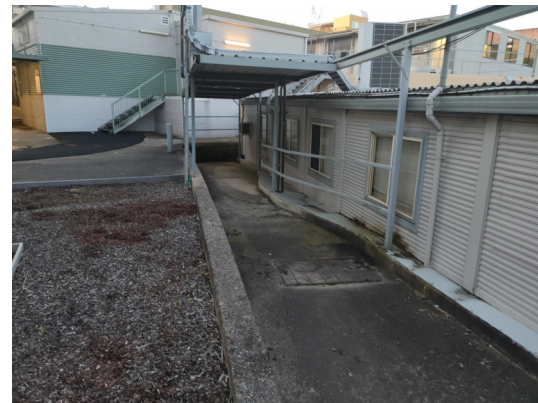
P11 PAVING TO BE DEMOLISHED IF ON GROUND, IF SUSPENDED RETAIN. RETAINING WALL TO LHS BE RETAINED. RHS TO BE DEMOLISHED TBC WITH CIVIL & STRUCTURAL ENGINEERS. CONFIRM WITH SERVICES ENGINEERS DRAWINGS THE SCOPE OF CABLE TRAY TERMINATION AND THEREFORE SUPPORT STRUCTURE DEMO.
